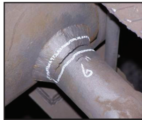
Tube Side Cracking
