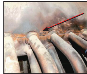
Seam Weld Cracking
